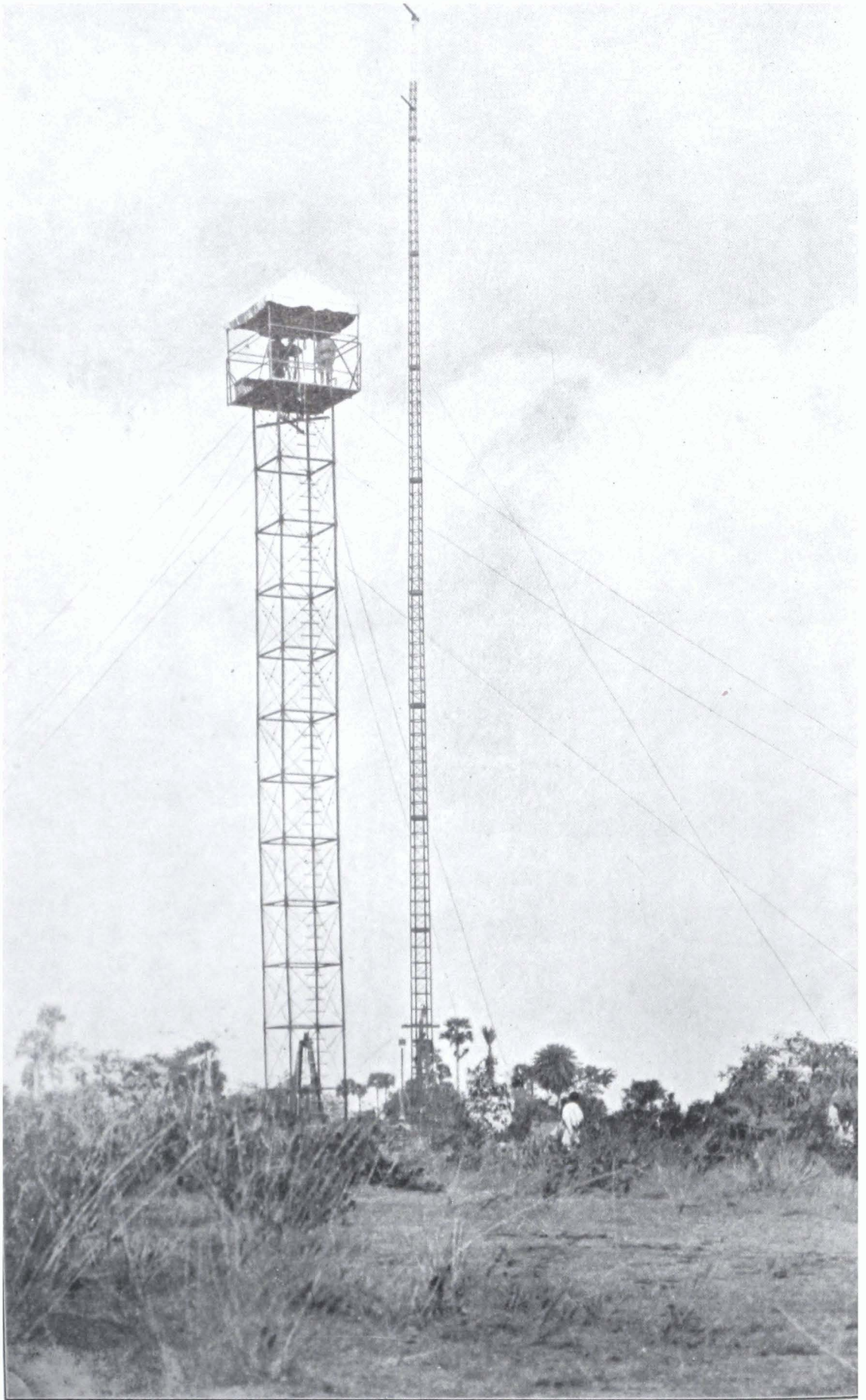
Kulamangalam Station, Madura Series, 1916-17. Height of instrument 67 feet. Height of signal 100 feet.
